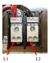
metal connection point to the hi-limit thermostat, cut back the shrink-wrap with a knife to expose the metal connection. A voltage reading around 120V should be indicated since this component is being fed by one leg of the electrical power coming off the terminal block. Perform this step on the bottom of each hi-limit thermostat then again on the top of each hi-limit thermostat.
