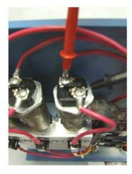
With the hot water tap opened and the temperature setting to the maximum, place one probe on one screw and the other probe on the other screw within the same element. You should be getting a reading of 220 + volts. Check all 3 elements and write down the voltage.
