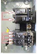
The **QUAD** breaker has four positions, the 2 OUTSIDE is 1 breaker and the 2 inside is another. Make sure you have 1 set of cables that are taped to gether **RED/BLACK** on the outside and the other **RED/BLACK** set that are taped together on the inside
