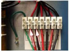
Now go ahead and follow the same steps, but this time measuring the TOP Screws. Write down the Voltage.
