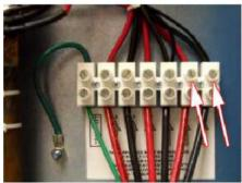
You should get a voltage reading when you measure across the screws in the 220 +. If you have NO READING at the bottom screws, make sure the breakers at the service panel and the main panel have been turned on.
