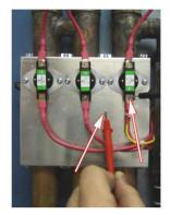
Test each thermostat both at the bottom section first, then the top section to make sure current is flowing through the thermostat.
